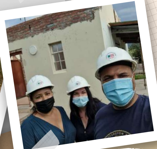
Sheraaz Ismail, Fatima Borez and Petro van Rhyin from Eco-Tourism and Access recently visited the construction site at Grootvadersbosch. The upgraded camping site is a very exciting new tourism development all campers can look forward to.
