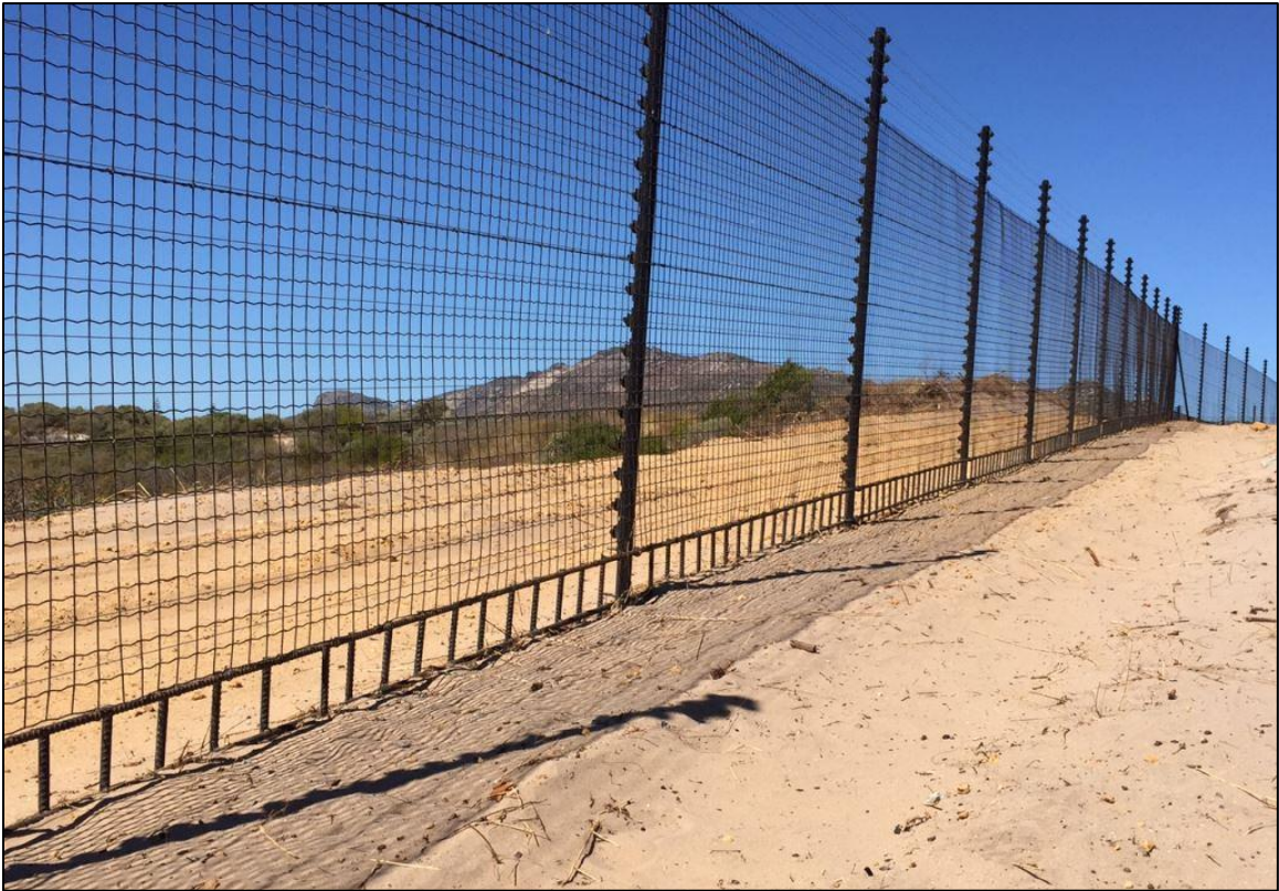
Figure 3. A fence designed to facilitate the movement of small animals between properties. This option could be considered where necessary. The gaps at the base of the fence must not be larger than 80mm to prevent use by baboons.
